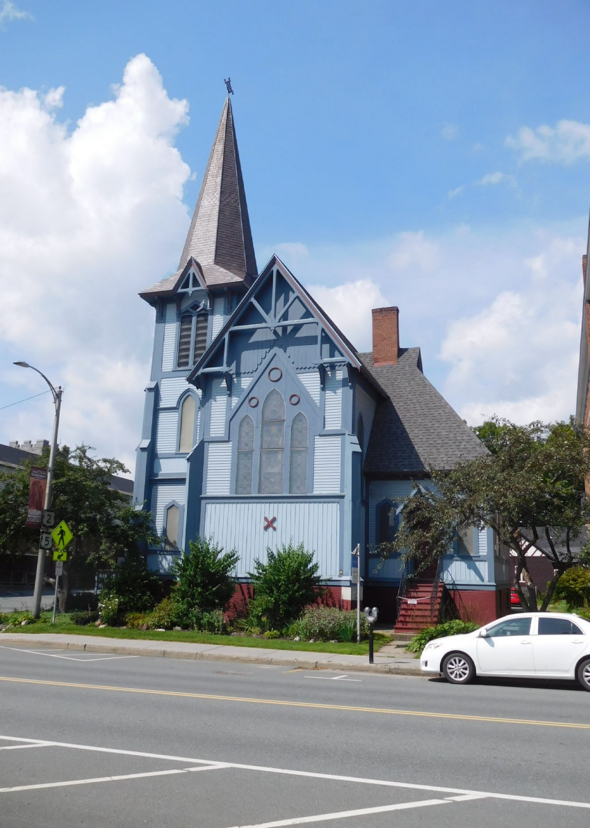
St. Andrew's Episcopal Church, St. Johnsbury
